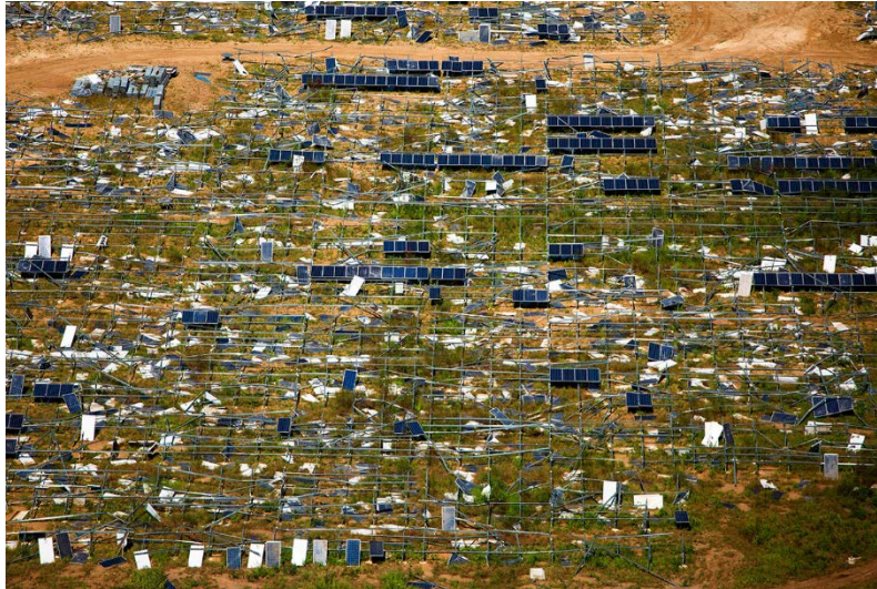
Figure 2. Broken solar panels in Humacao
